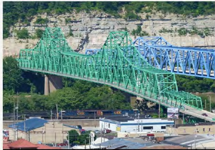
2006 Ashland, KY Bridges
