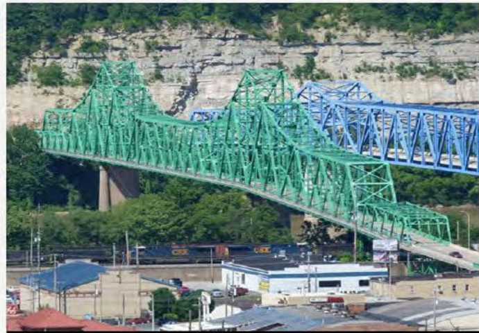
2006 Ashland, KY Bridges
