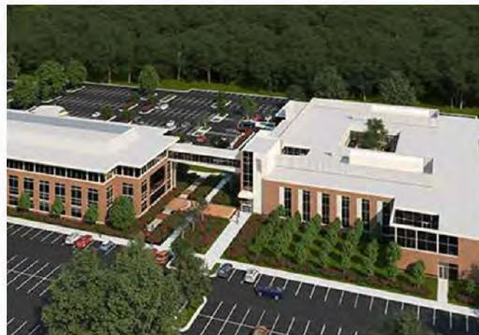
2020 Upper Chesapeake Hospital
